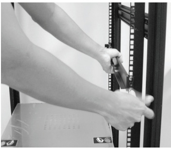
1. Secure the side rails to the rack.
